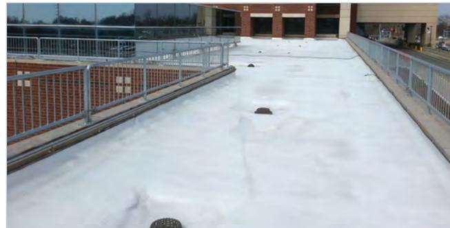
One of the most difficult aspects of this roofing project was the drainage. On top of requiring new slope, the roof had over 150 penetrations, most of these in the form of roof drains. Foam was the best tool available with regard to guiding water to the drains, and then creating a smooth, water-tight seal at the drains.
