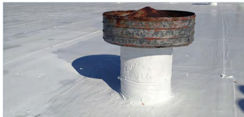
The previous roofing system, a smooth-surface built-up roof, had severe wear and tear around all protrusions and building edges. These areas were treated with a three-course silicone system that consisted of coating-fabric-coating to ensure a water-tight seal.
