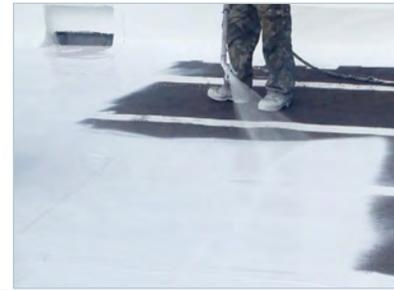
All protrusions in the roof were treated with a three-course silicone system that consisted of coating-fabric-coating and received coating on the entire fixture. This ensured a watertight seal where the old system was vulnerable to leaks.
