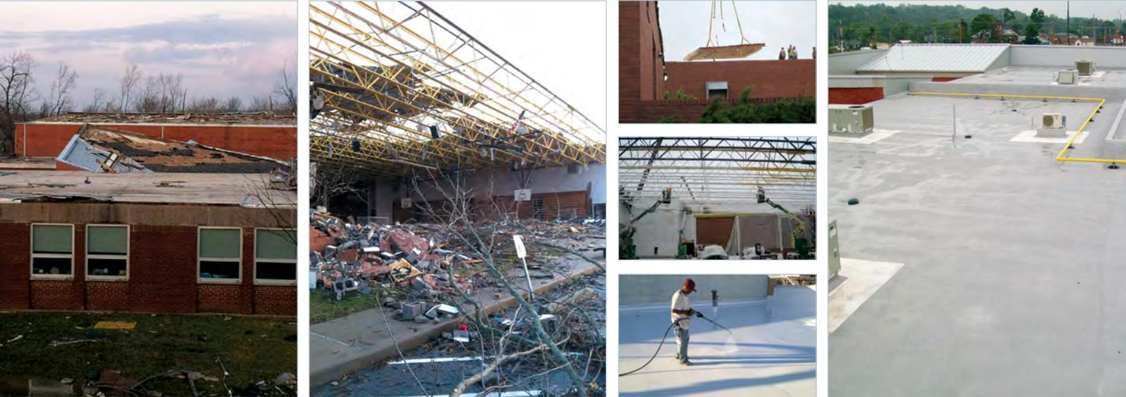
Tornado damage to the Henryville school buildings was extensive, with entire portions of the buildings demolished. The tedious process of removing damaged sections and rebuilding occurred around the clock. Within 6 months the entire structure had been rebuilt for the start of the next school year. The new roofing system takes advantage of cutting edge technology and is now sustainable and energy efficient.
